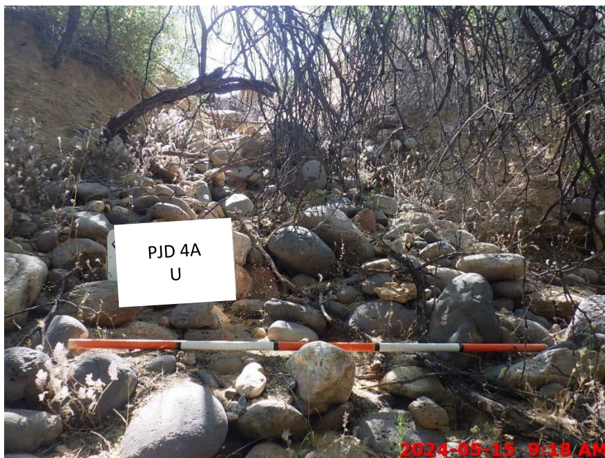
View of PJD 4A looking upstream (east) toward fill area for SR 96 realignment near MP 11.03.
