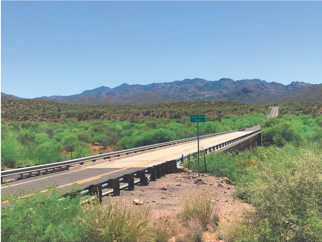
Figure 3: View of the existing Santa Maria Bridge looking to the southwest
