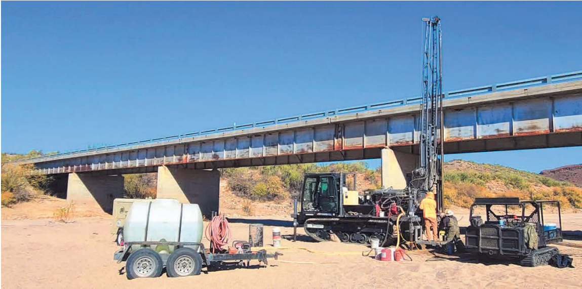
Figure 5: Subsurface investigation, boring B-3, on December 6 th , 2024
