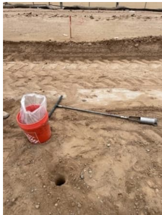
Boring R-106, Overhead Utility, Hand Auger
