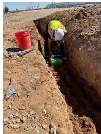
Typical, Nuclear Density Testing
