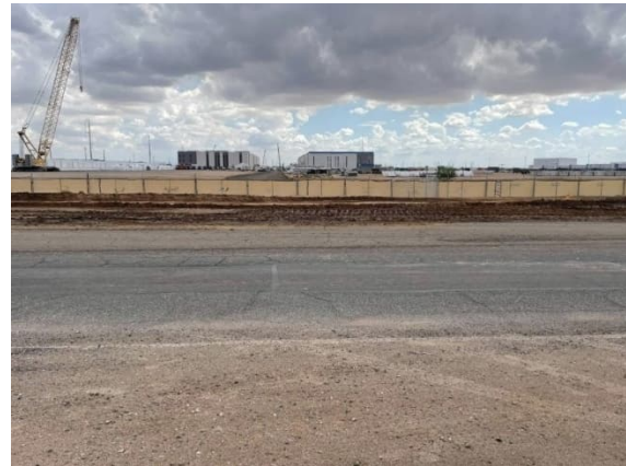
Near Boring R-106, Facing East, Reems Rd
