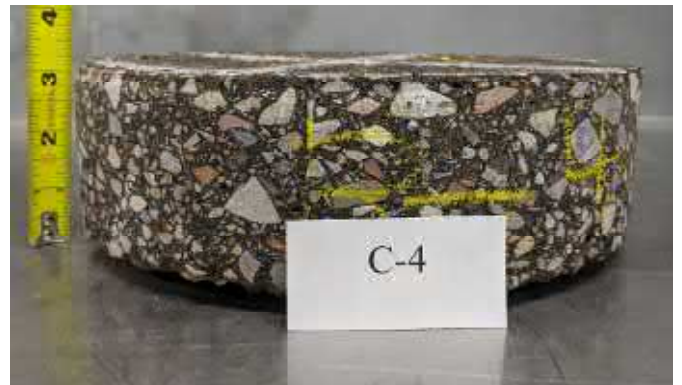
Photo No. 4: View of Core 4; B-4
