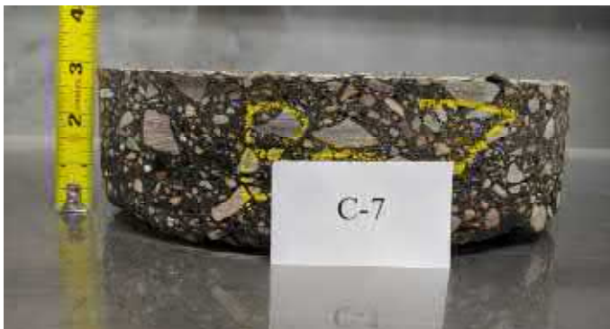
Photo No. 7: View of Core 7; B-7
