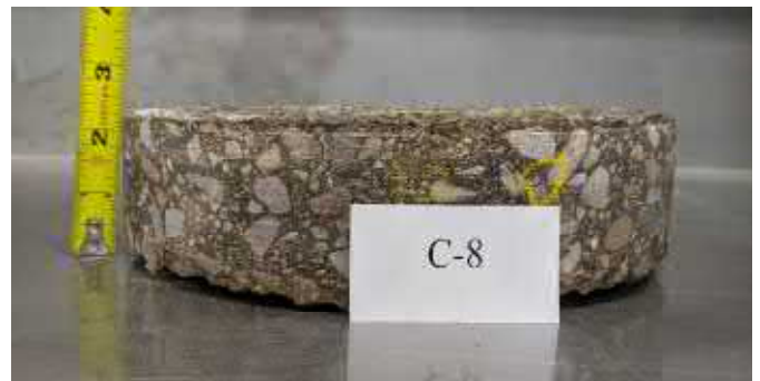
Photo No. 8: View of Core 8; B-8
