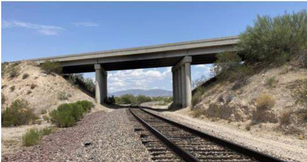
Figure 3: View of the existing Rail Crossing Bridge looking to the north
