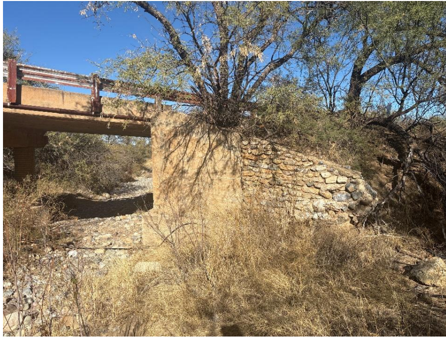
Figure 2. Florida Canyon Wash Bridge northeastern wingwall
