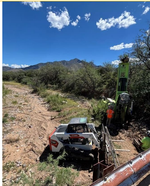
View of Sonic Rig on MB1
