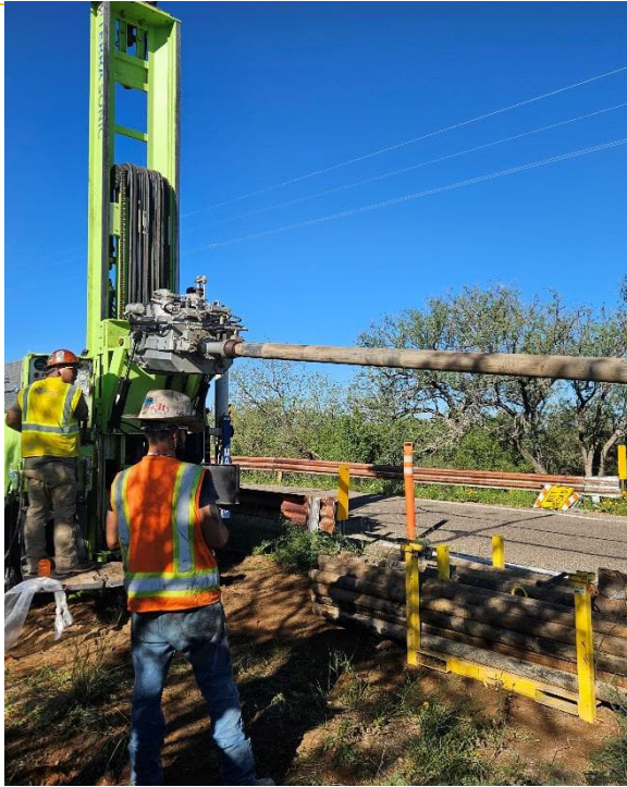
Setting up Sonic Rig on MB2
