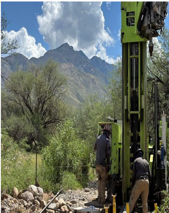
View of Sonic Rig on FB1
